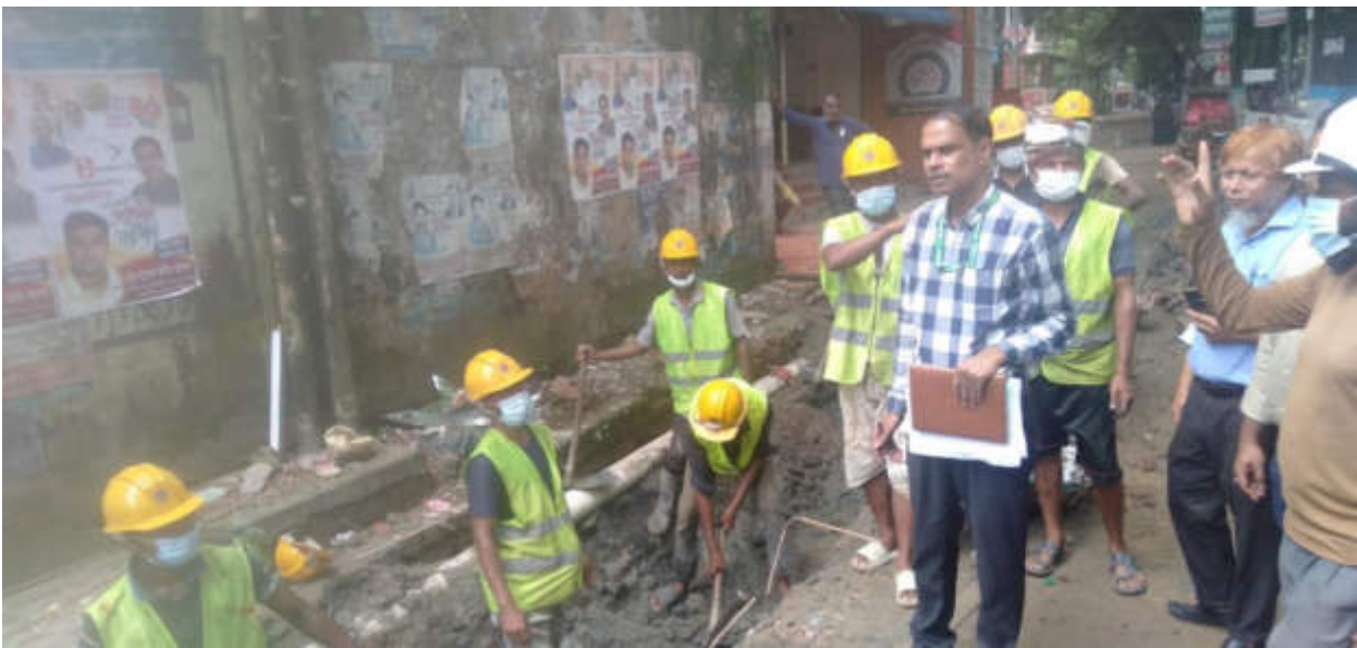
Workers are busy in a Road work in Brahmanbaria Pourashava area wearing PPE
